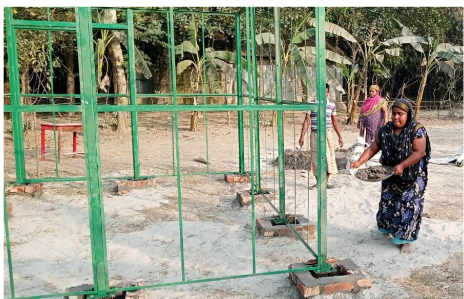
Community based drying dome under construction
